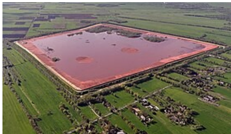
Figure 3. Bauxite residue pond near Stade (Germany) [3].
